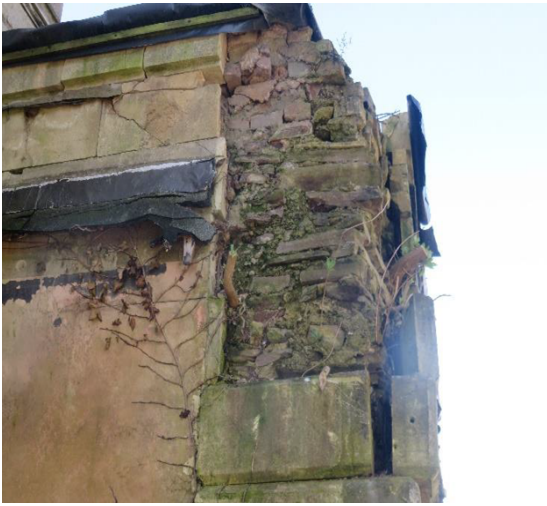
Photographs 4 and 5: Buddleia roots growing through gaps in the masonry of the building.
