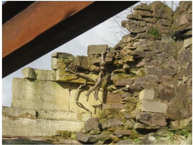
Photographs 4 and 5: Buddleia roots growing through gaps in the masonry of the building.
